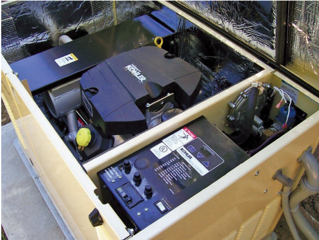
FIGURE 32-4 A natural gas-fueled generator. (Courtesy of Kohler Power Systems)
