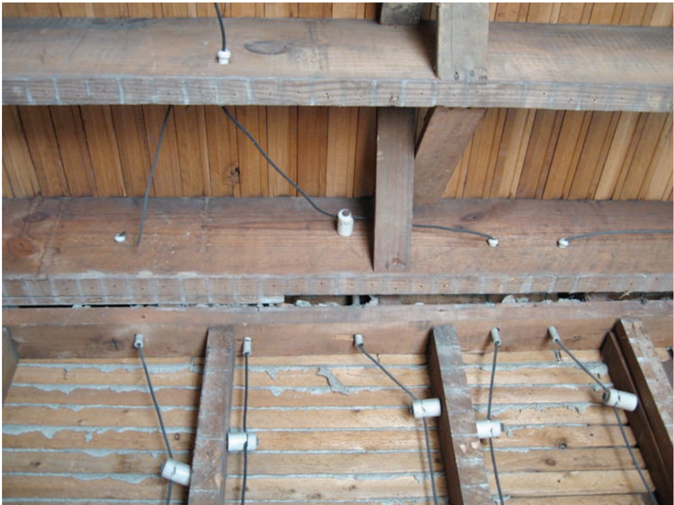
FIGURE 4-5 Photograph of a typical knob-and-tube wiring from the 1930s. (Delmar/Cengage Learning)
