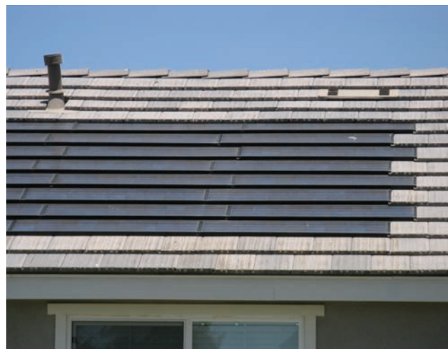
FIGURE 33-5 Building-integrated photovoltaic roof tiles. (Delmar/Cengage Learning)
