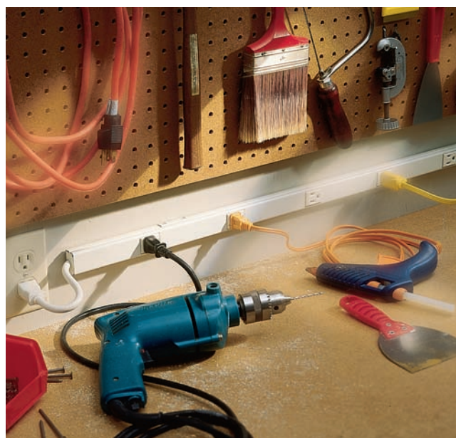
FIGURE 18-18 A cord-connected, prewired multioutlet assembly installed above a workbench. (Courtesy of The Wiremold Company)
